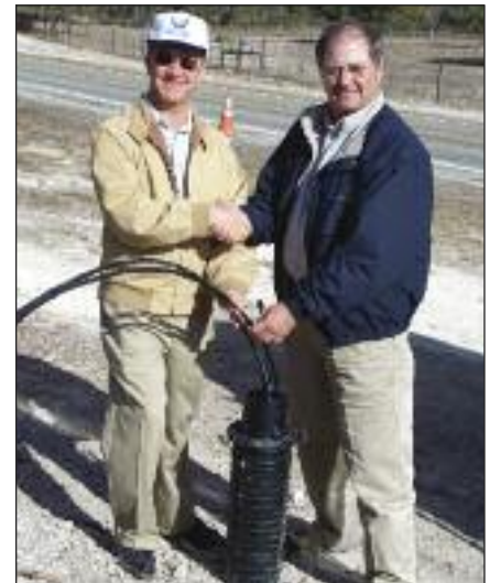
SWTTC General Manager Gary Gilmer and HCTC General Manager Delbert Wilson (l to r) signify "the linking" of their respective company cable facilities in order to provide more efficient transportation of data required of broadband and other state-of-art communications services.
